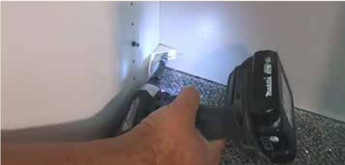
The Zip-It/Tornado anchor is a one-piece self drilling anchor designed specifically for use in gypsum wallboard.
